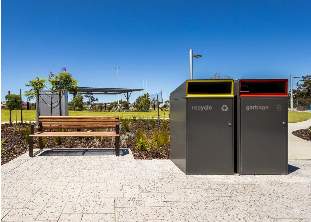
Subiaco East Redevelopment, Perth, WA, specified by UDLA. Escola Bin Enclosure (WBE-E240) in Woodland Grey and Rectangle opening insert in Brilliant Yellow and Lobster Red.
